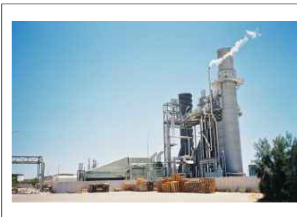
Combined cycle co-generation site
